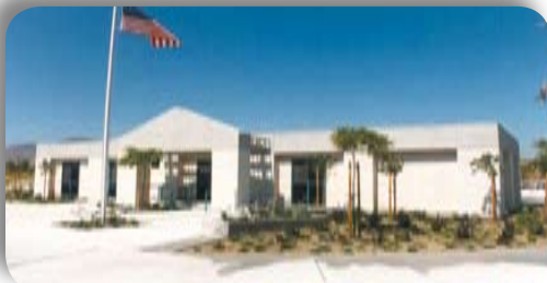
24' x 60 Fire Station
